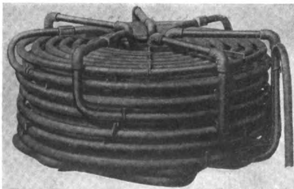
White Generator, Showing Coil Connections.
